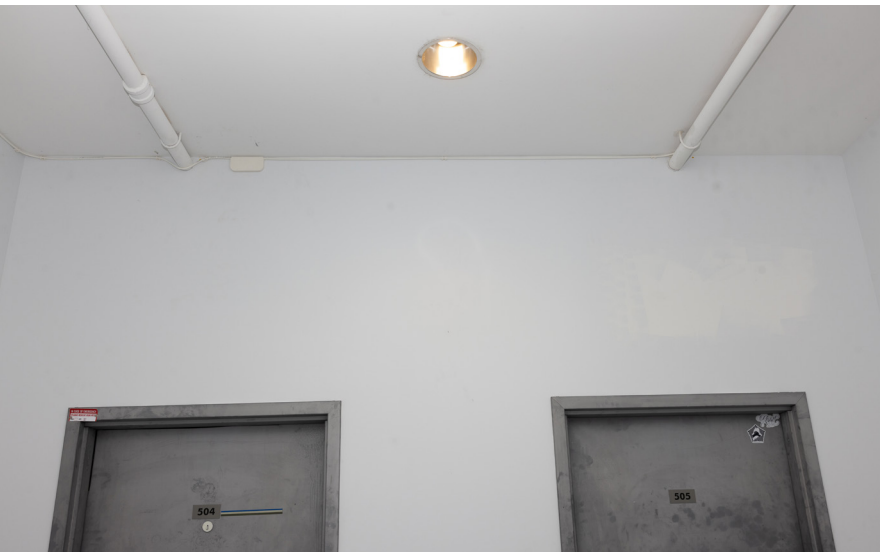
The PPC QuikPass™ solution is installed across the ceilings of the MDU building's hallways.
